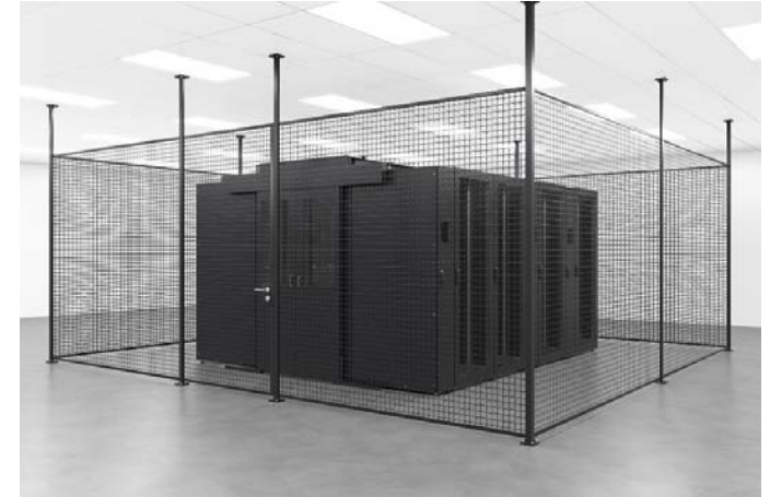
Rack Space 47- Caged
